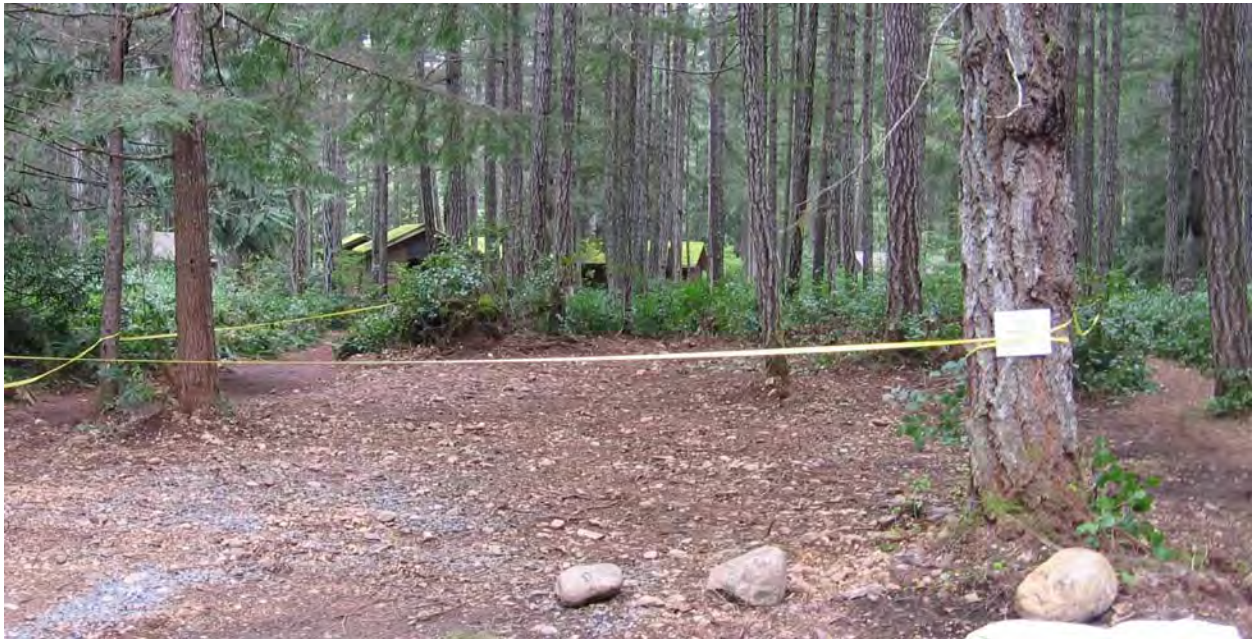
Figure 10a. Septic field area before restoration.
