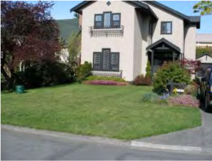
Before renovation (April 2011)
